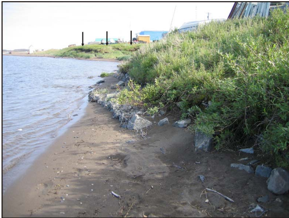
Figure 7. Erosion of sandy alluvial terrace sediments along Kugluktuk's northern shore. Gabion baskets (foreground) that were installed to reduce erosion are now being undercut and/or destabilized by wave-induced erosion. Wave-induced undercutting of vegetated slopes seen in the background (marked by arrows) has resulted in slumping of sediments along the base of the active layer. Exposure of underlying frozen sediments along cracks will lead to further erosion. (photo, I.R. Smith)
