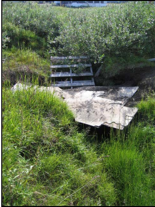
Figure 8. Stream erosion atop alluvial terrace sediments beside the sea shore, Kugluktuk, Nunavut. Channelling of meltwater and rainwater from community through an unarmoured channel has resulted in physical erosion and incision. Incision of the channel has also likely led to melting of underlying permafrost, resulting in thermal erosion, and enhanced over-deepening of the channel. Slumping of sediments along channel margins points to ongoing instability and lateral propagation of the channel margins. (photo, I.R. Smith)
