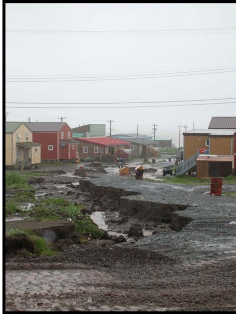
Figure 9. Erosion of Kugluktuk streets as a result of the extreme July 20-21, 2007, storm event (170.7 mm). [source: photo by J.Prno, 2007; climate data from Environment Canada's online National Climate and Information Archive]
